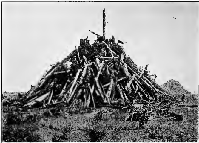
Fig. 53. Stumps Piled Around Gin Pole in Clearing with a Donkey Engine
